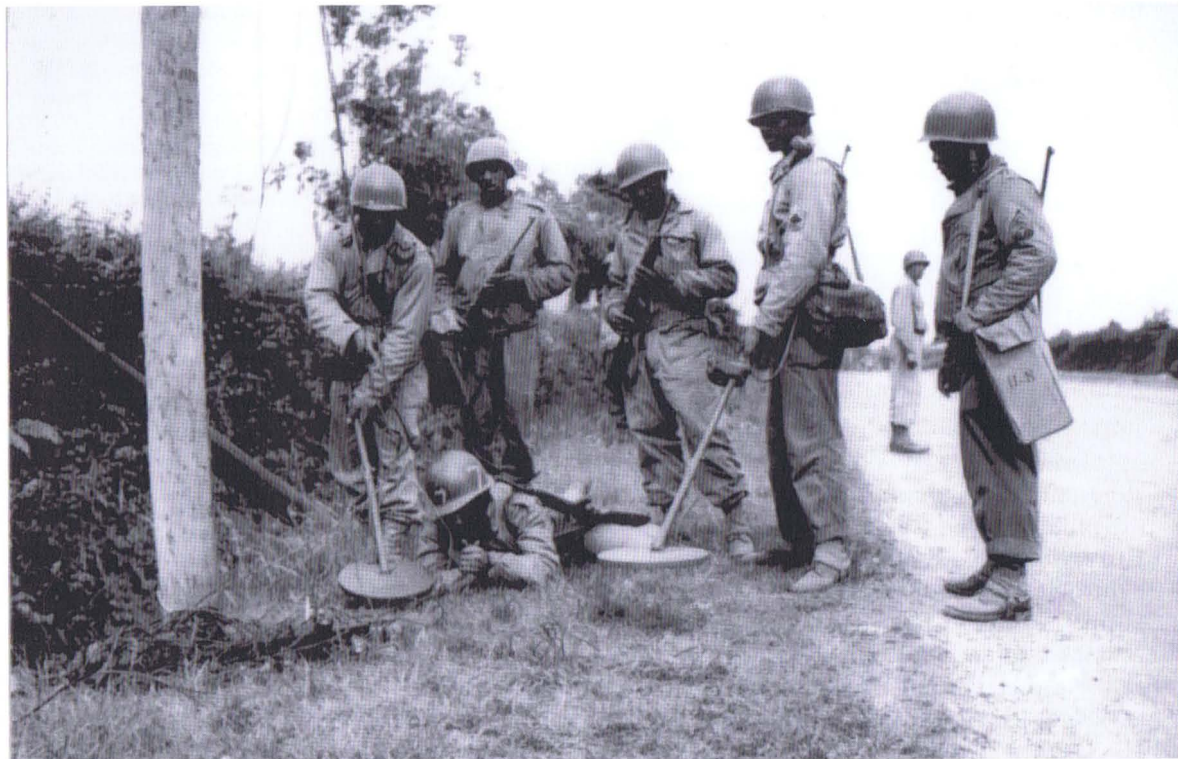
A posed group of African American US Army engineers demonstrate the use of the SCR-625 mine detector. These were often used in pairs so as to sweep more rapidly a path of vehicle width. A man probing by hand would precisely locate and examine the mine discovered by the detector. Road verges were a favorite site for mines and booby traps, to catch unwary drivers who ran a wheel off the road when passing other traffic or speeding at a bend, or personnel, who habitually walked up each side of a road rather than on it.
